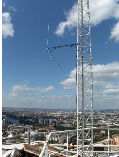
FIGURE 4 DRM ground plane antenna on top of the Tour Pleyel
