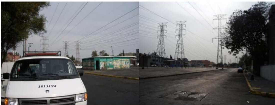
FIGURE 31 Location environment of high voltage tower test
